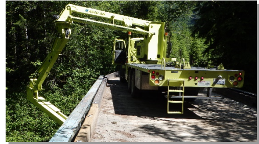
Figure 1.1: An Under Bridge Inspection Truck at a timber and steel bridge in King County, Washington.
